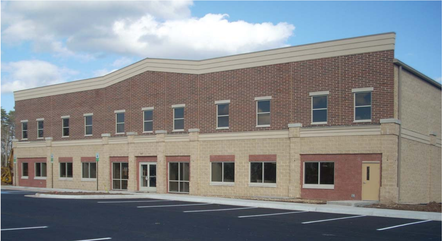
D.A Foster's newly constructed office/warehouse building.
