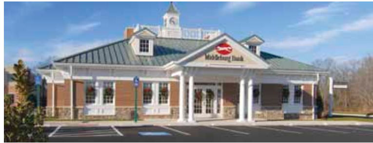
Middleburg Bank's newly completed branch.
