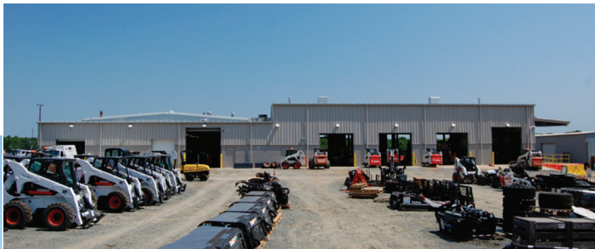
Bobcat of Virginia addition, rear view
